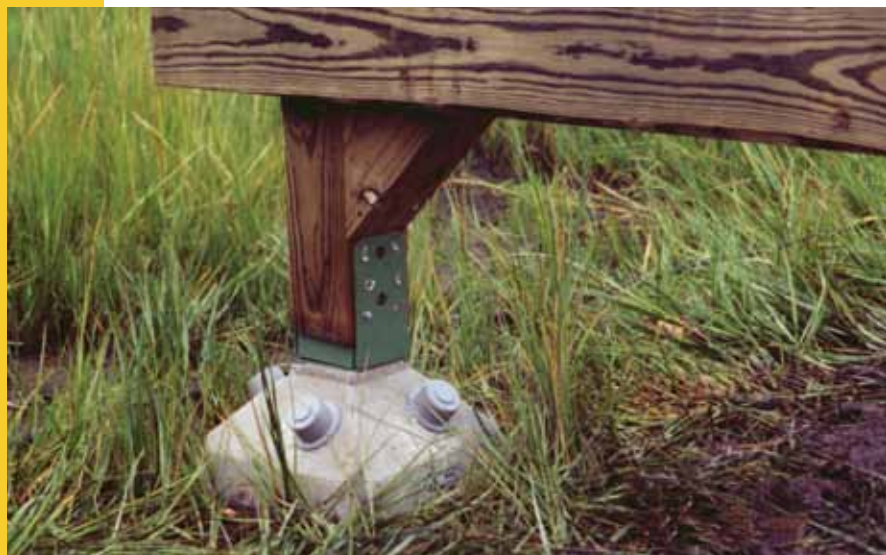
Engineered Diamond Pier foundations fit into any low-impact strategy, bringing an environmentally friendly solution to a wide variety of construction sites.
