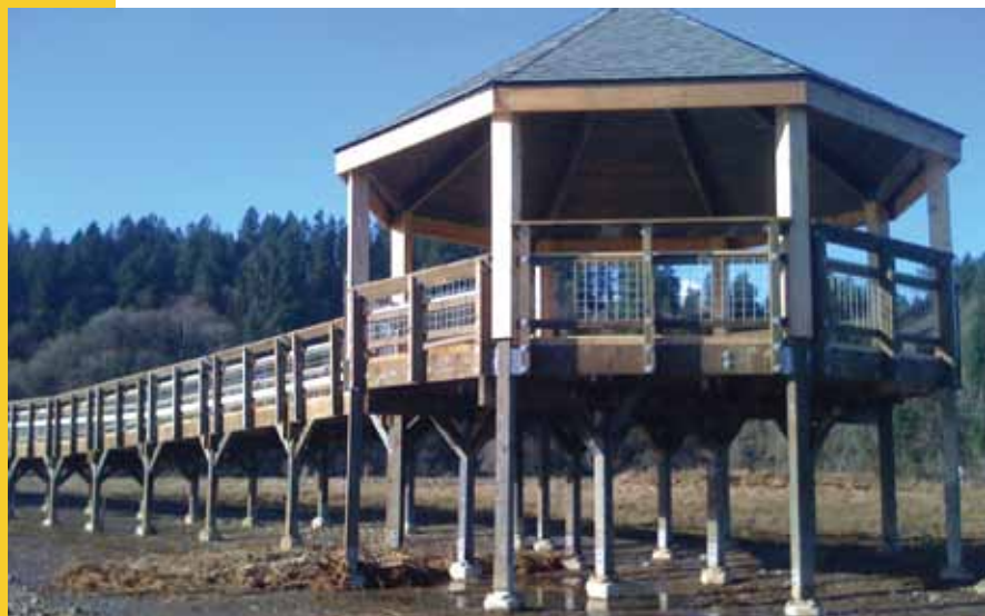
High strength concrete heads interlocked with driven steel pin clusters provide resilient, durable foundations for boardwalks, bridges pavilions, and overlooks.
