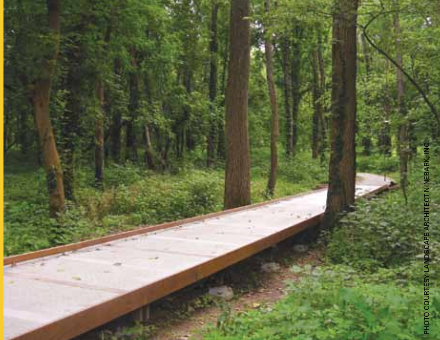
Diamond Piers allowed construction of this walkway with minimal site disturbance in this historic forest at the Indianapolis Art Museum Virginia B. Fairbanks Art and Nature Park.
